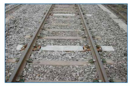
Due to the concrete and corrosion-free carbon reinforcement, the sleeper body will not suffer corrosion due to stray currents from DC conductor rail or traction bonds.
