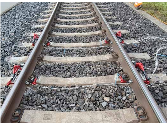
Track measurements under operating conditions
